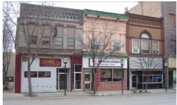
This cluster of hospitality businesses would benefit from a coordinated façade improvement package. Added income from upper floor residences could provide cash flow to pay for business improvements.
