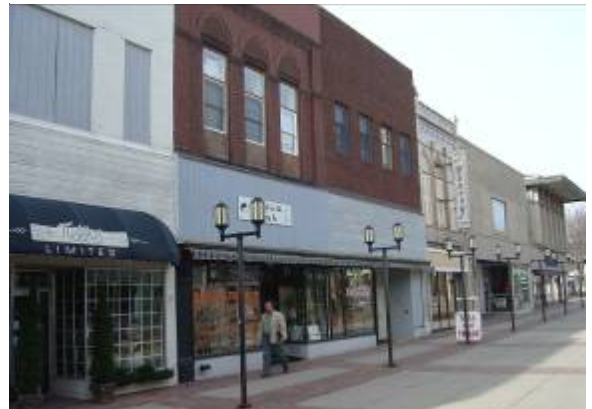
Upper floor uses along Federal Plaza should include housing, office, and dining. Think balcony.
